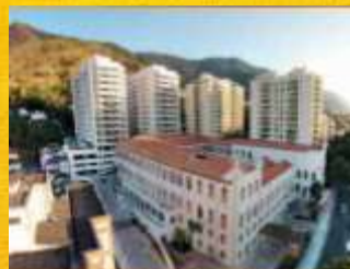
Atrium Residences & Lofts Rua Dona Pízzuto, 481 - Tijuca
